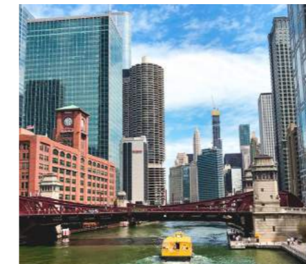
DC Chicago, 350 E CERMAK RD Floor 7 Room TECH
